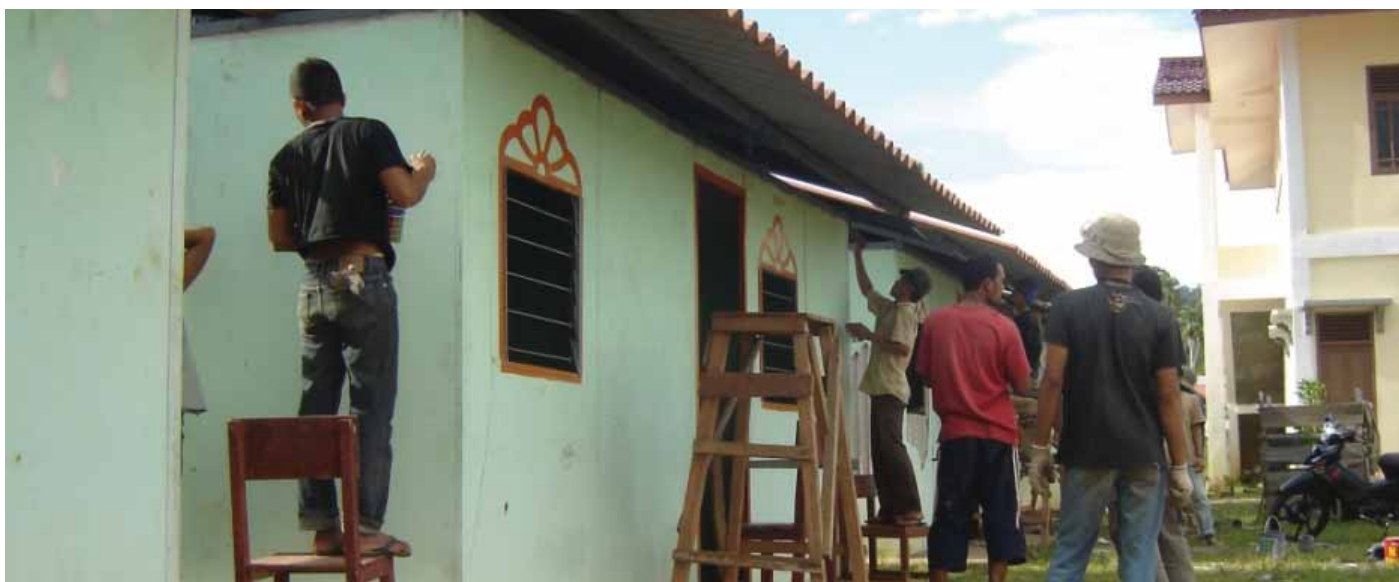
Pesantren Budi, Janguet village, Aceh Jaya district during construction maintenance work
